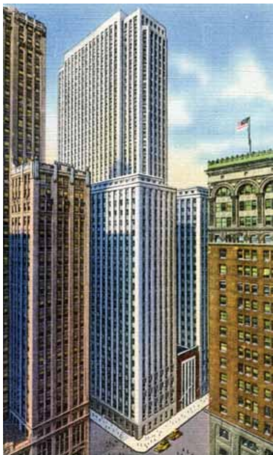
Field Building , 135 S. LaSalle Street, Graham, Anderson, Probst, and White, 1934, view from southeast. (Contemporary postcard, collection of the author)
